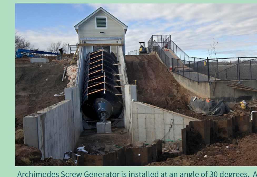
Archimedes Screw Generator is installed at an angle of 30 degrees. ASG has three blades with a runner diameter of 139.75 inches. The intake is hydraulically controlled by a sluice-gate to ensure a run-of-river flow design.
